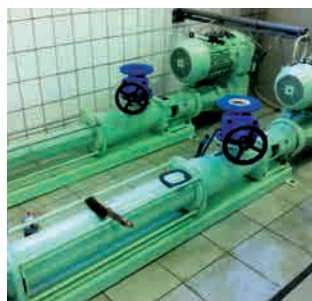
Conveyance of thin slurry: KL50S progressive cavity pump
