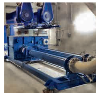
Conveyance of dewatered sewage sludge: KL80RQ110.4+110.4 Progressive cavity pump
