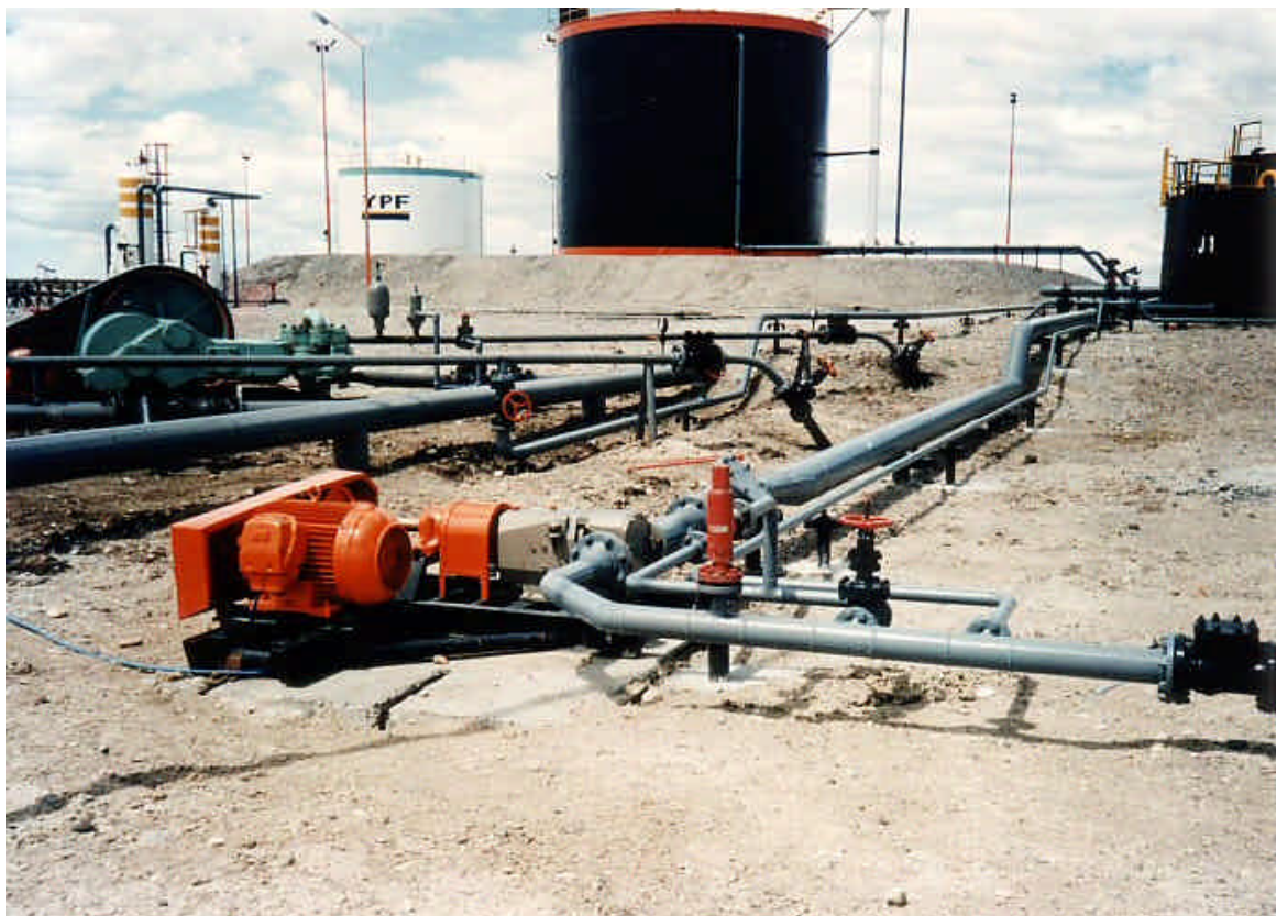
Series D6 pump handling crude oil in Argentina
