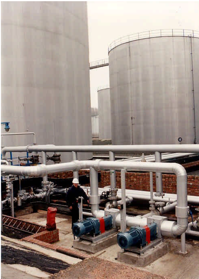
Series D6 pump at UK oil terminal used to feed a separator to remove hydrocarbon residues from surface water
